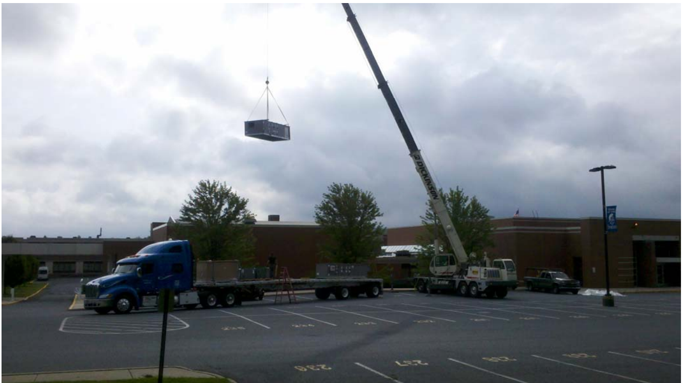
Photo of one of three air handlers being placed on the High School Roof in conjunction with HVAC project
